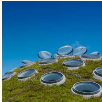
Heating and Cooling
